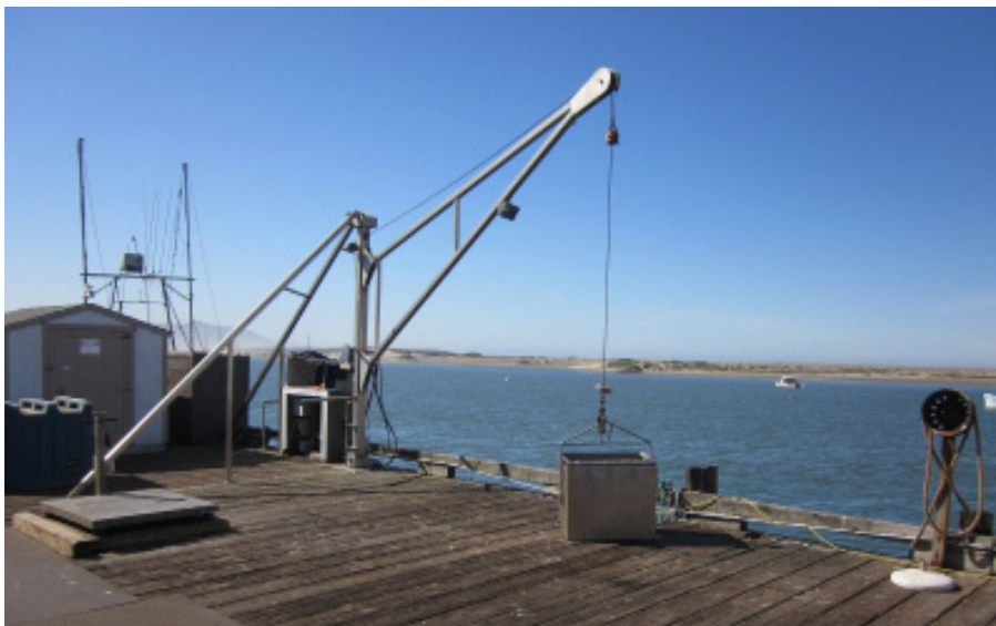
Photo: 2,000 pound stainless steel offloading hoist at the 1099 Embarcadero facility.
