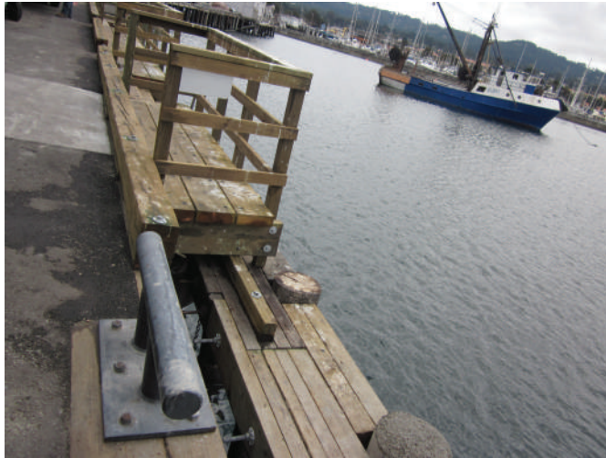
This cleat, on the south side of Municipal Wharf II, would cost approximately $3,000 provided by an outside vendor. It was fabricated and installed by the Harbor Division crew for a little over $400.
