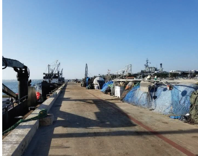
Fig 3.13 – Gear storage on G Street Pier – looking towards G Street Mole. Taken October 9, 2017
