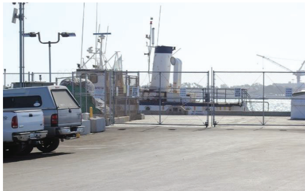
Fig 3.7 - Newly installed chain-linked gate at head of G Street Pier. Taken October 9, 2017
