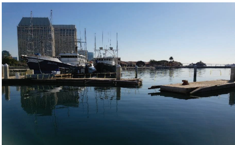
Fig 3.5 – Tuna Harbor dock damage. Taken - December 19, 2017
