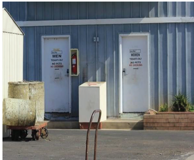
Fig 3.36 - On-property restrooms at Driscoll's Wharf. Taken October 9, 2017.
