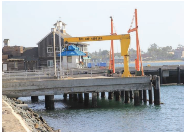
Fig 3.19 - Offloading cranes located in Tuna Harbor. Taken October 9, 2017
