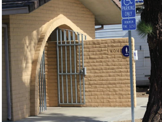
Fig 3.37 - Public restroom adjacent to Driscoll's Wharf. Taken October 9, 2017.
