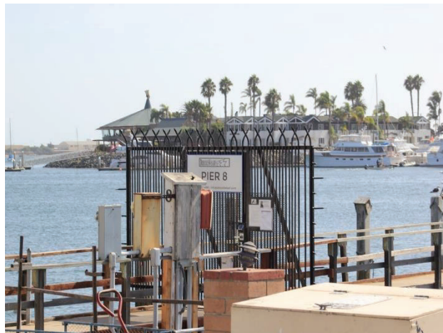
Fig 3.34 - Security gate atop Pier 8 at Driscoll's Wharf. Taken October 9, 2017.
