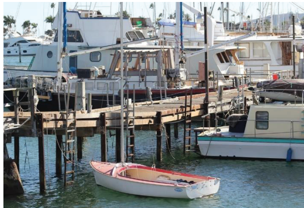
Fig 3.29 – Ladders utilized to get on and off a vessel berthed at Driscoll's Wharf. Taken September 25, 2017.
