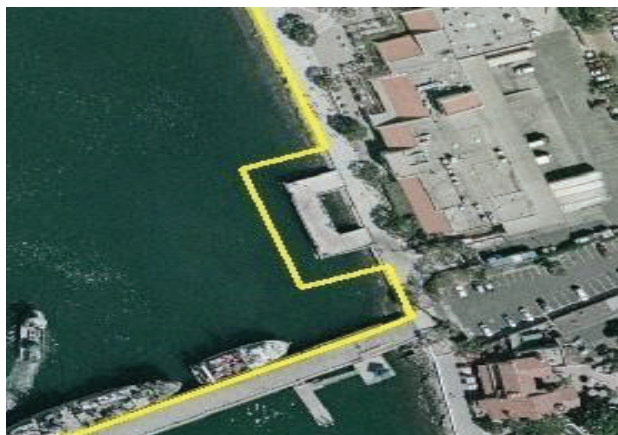
Fig 3.18 – Location of offloading cranes in Tuna Harbor
